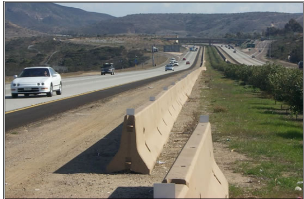
Figure 26: Median Barrier with gap. Caltrans photo.
