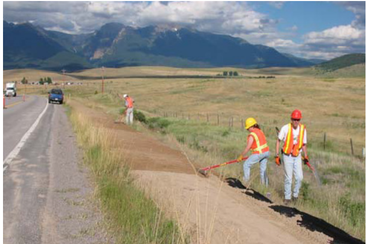
Figure 11: Installation of raked soil beds adjacent to US-93 in Montana (Montana DOT, 2006).
